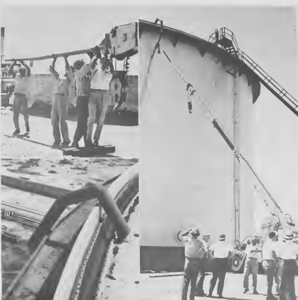
NEW WAY to reach the tops of the tallest tanks in the field is demonstrated by this attachment, denominated by the manufacturer as a hydraulic crane. It allows quick placing of a diaphragm seal, coal to install arbores on the hydraulic crane. It is permitted to place one tube of support or a curved pipe rapidly on the pipe arbores and to work six feet above the level of the ground.
